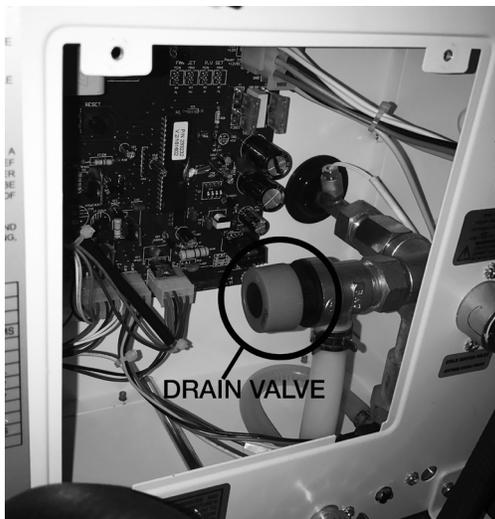
6. Turn drain valve knob clockwise to drain and then clockwise again to close.
